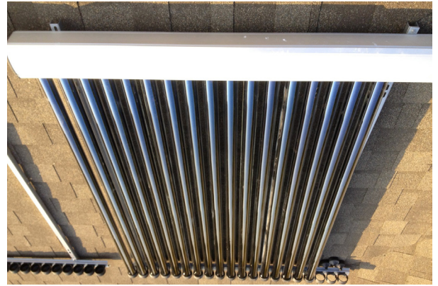
This array of vacuum solar tubes is able to generate temperatures of over 100°C on sunny days, even when outdoor temperatures are below freezing. Photo credit: Reiner Hoyer
