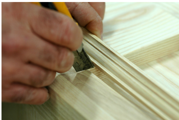
A utility knife is the best tool for marking trim to length for accurate cutting. Photo credit: Steve Maxwell
