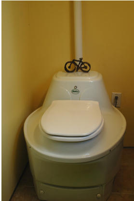
Composting Toilet Photo credit: Steve Maxwell
