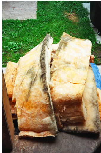
The black and grey patches on this fiberglass insulation are the telltale signs of air infiltration, wintertime condensation and mold growth.
